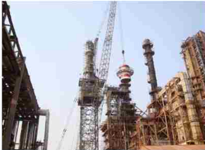
Maintenance, Shut Down / Revamp
