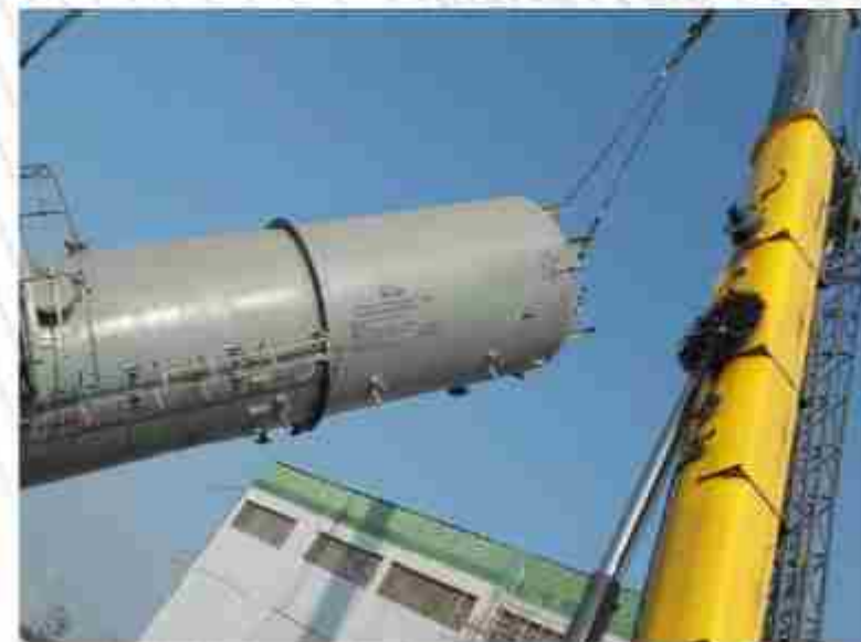
Fabrication & Erection of Equipments
