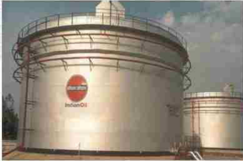
Cone / Dome Roof Tanks
